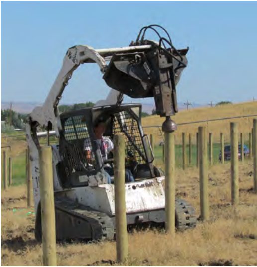
Figure 4.10 Line post installation in a vineyard
