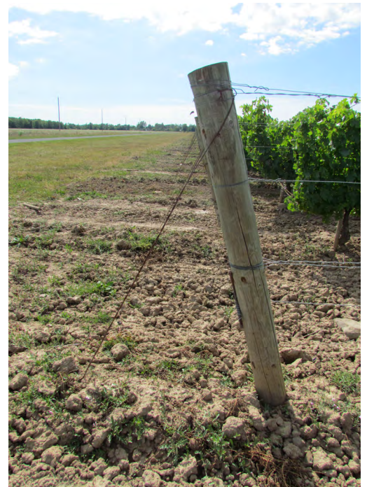
Figure 4.16 Inclined end post with anchor
