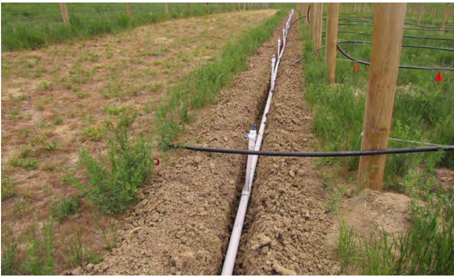
Figure 4.17 Installation of a drip irrigation main line in the vineyard
