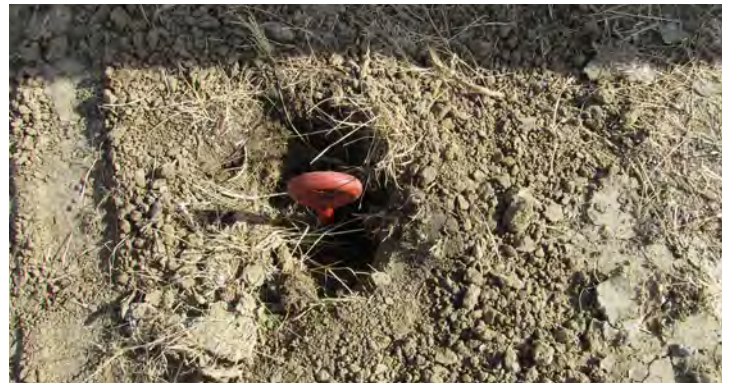
Figure 4.14 Installed earth anchor
