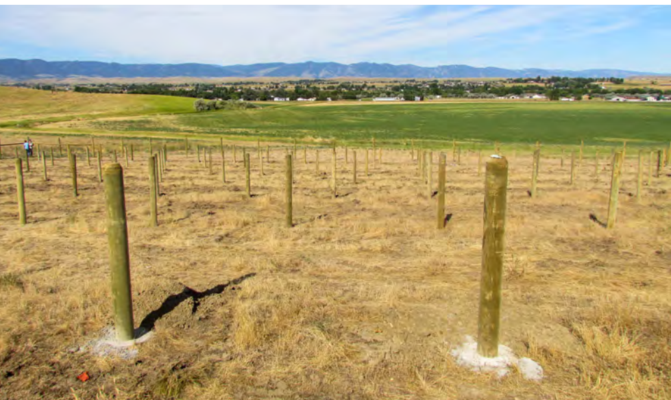
Figure 4.9 Line post installation in a vineyard
