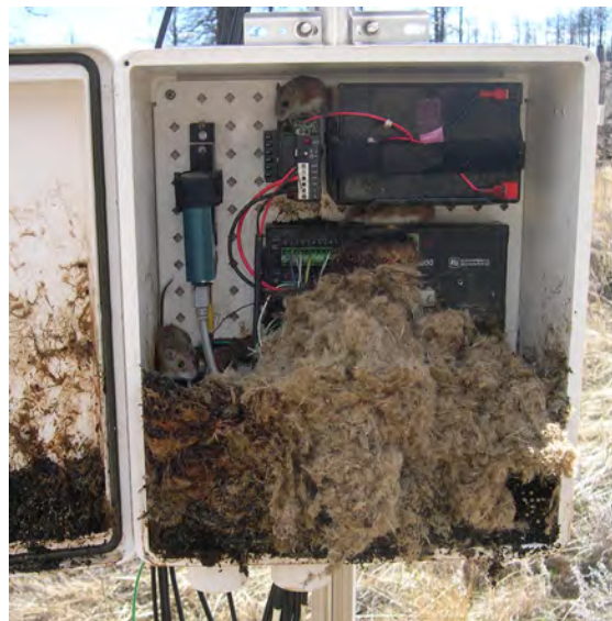
Figure 45. A , During the winter of 2013–2014, mice gained access through an opening in the bottom of the weather station at RRS. In spring 2014, co-author Steve Williams discovered a substantial nest and droppings in the box, along with three live mice. B , Lead author Mollie Herget (pictured, at left), and summer intern Tunsisa Hurisso (right) removed the materials from the box and then did a thorough cleaning; however, it was discovered that the mice caused damage to panel wiring and other electronic equipment, leaving the station inoperable. As discussed in the text and Figure 49 caption, repairs were made in fall 2017. (Photo by S. Williams)
