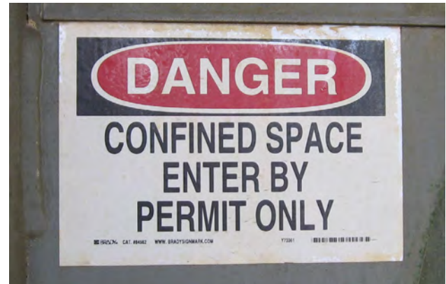
Figure 5-6. Sign posted next to a cylinder door to warn workers that the cylinder is a permit-required confined space.
