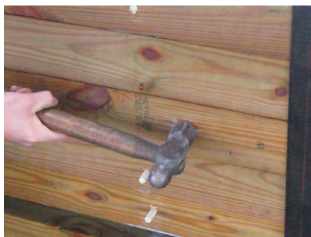
Figure 9-3. Treated wood plugs (left) are hammered into holes left from taking wood samples (right).
