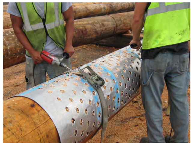
Figure 6-4. Radial drilling groundline area of utility pole prior to pressure treatment.
