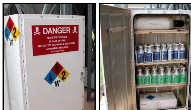
Figure 6: The photos above show the outside and inside of a fumigant storage locker located next to grain silos where they will be used. You must secure pesticides storage areas for any pesticide, but it's especially important for fumigants because of their high toxicity. Proper warning signs and placards are important and often prescribed by the label and sometimes by state regulations. Make sure you are following all guide- lines. Photo credits: © J. Ples Spradley, pesticidepics.org at Virginia Tech.
