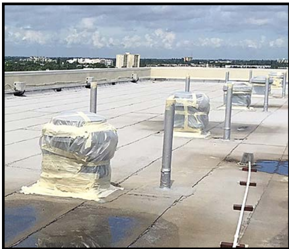
Figure 3: Part of a large sealed fumigation job is shown above on the left. Note all the roof vents are heavily sealed. While necessary in cases where enclosing the whole building under a tarp is not practical, sealing can be labor intensive. Make sure to seal all places where fumigant gas could escape. Use gas-impervious tape, and in the case of entryways, such as that on the right, placard and secure the door from entry. (Photos © Douglas Products).
