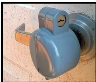
Figure 2: You might need to use different kinds of locks to prevent entry to the fumigation site. Three examples of locks you can use include clam shell, key-way, and J-safe locks. Clam shell locks are designed to prevent use of the door or occupants' keys to unlock entrance doors.
