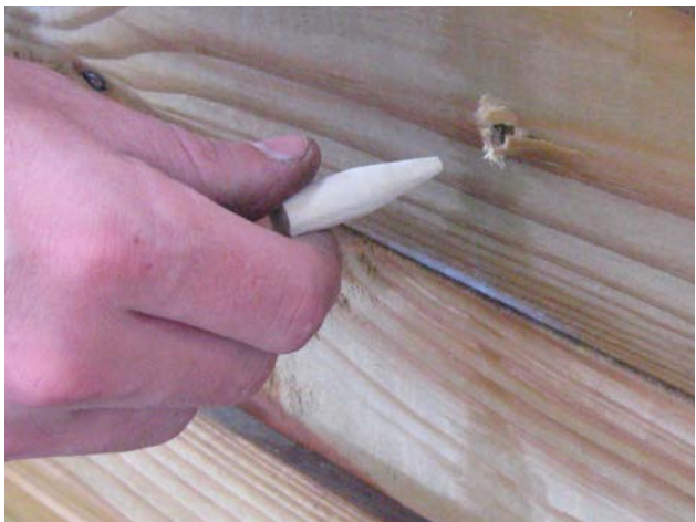
Figure 9-3. Treated wood plugs (left) are hammered into holes left from taking wood samples (right).
