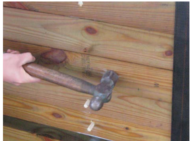
Figure 9-3. Treated wood plugs (left) are hammered into holes left from taking wood samples (right).
