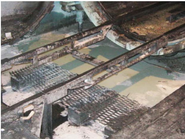
Figure 4-5. Tracks spanning over door pit from drip pad to cylinder.
