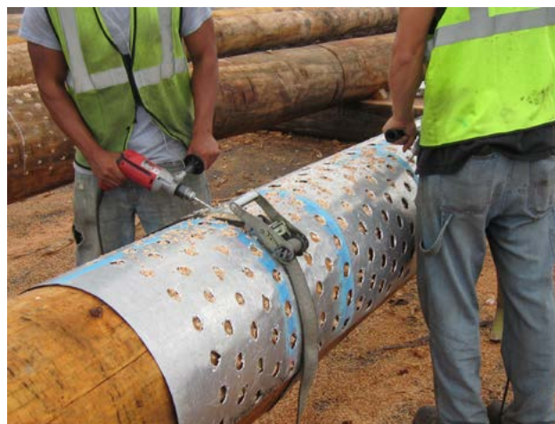
Figure 6-4. Radial drilling groundline area of utility pole prior to pressure treatment.
