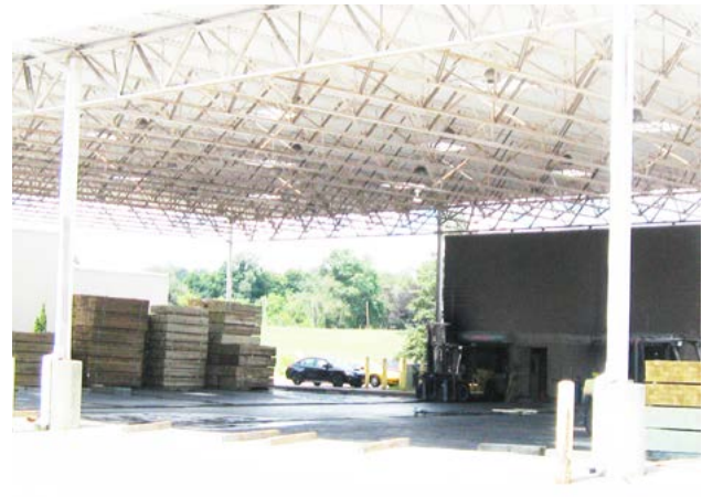
Figure 4-8. Covered drip pad
